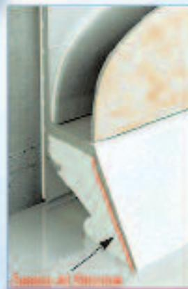
Each Cladseal strip has a green tape (the red line) applied to the inside face of the strip. Sealux-N silicone cannot bond to this tape after it cures. When joint movement occurs between the ledge and wall, the Sealux-N silicone simply releases off the green tape (under tension) and stretches to accommodate joint movement. All very simple!
